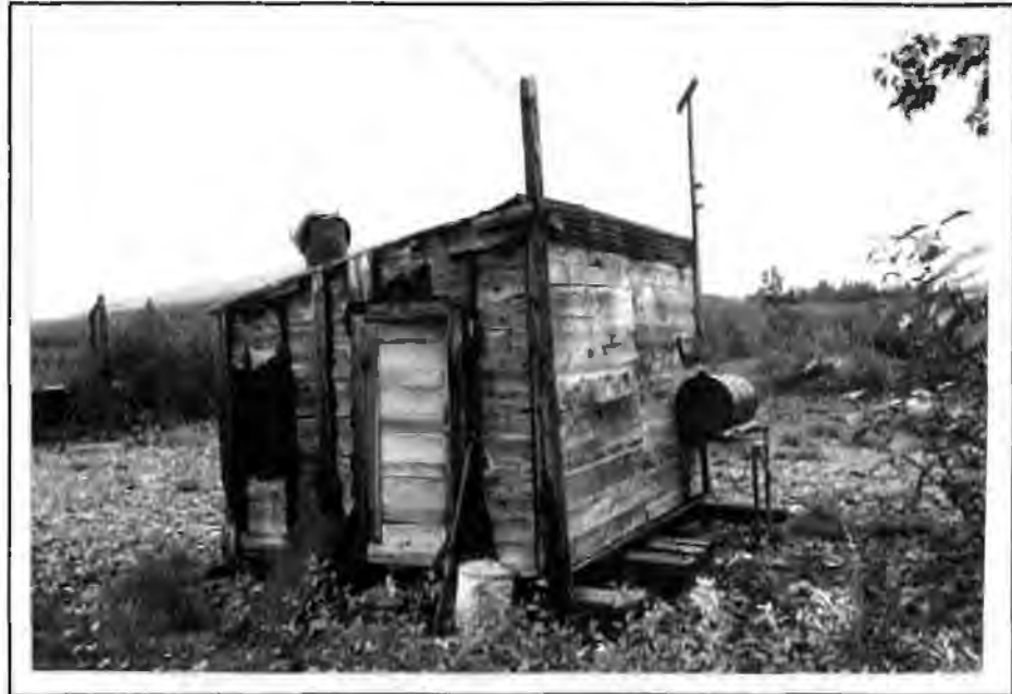
Figure 136. The Generator Shed, 1993. The view is looking northeast.
